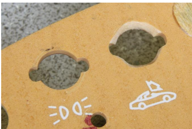
Figure 5: Unmodified (left) vs. beveled (right) bulb hole
